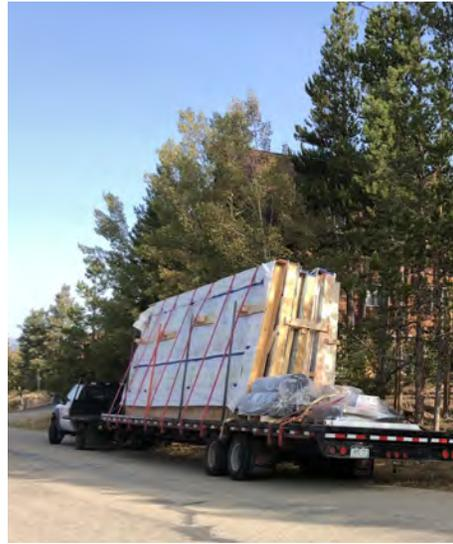
Figure 7: SPARC House panels on truck
