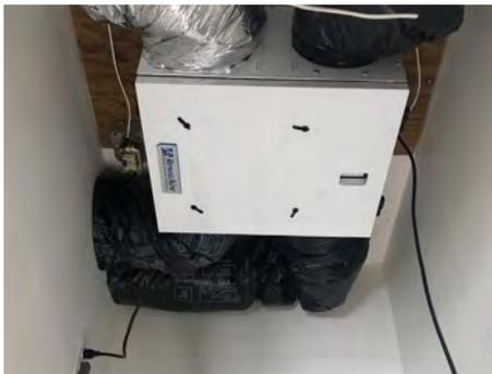
Figure 13: ERV on ceiling of mech room
