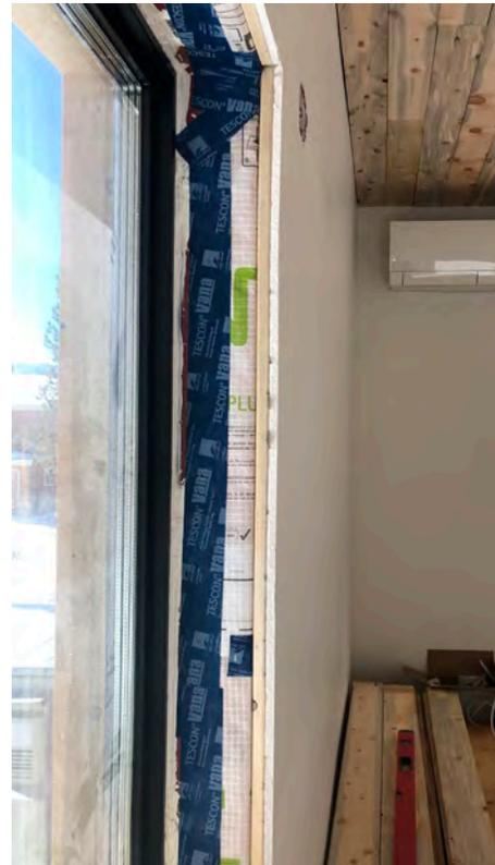
Figure 10: In-set window and wall layers
