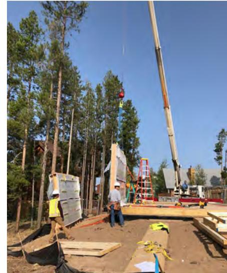
Figure 8: Crane placing panel on floor box
