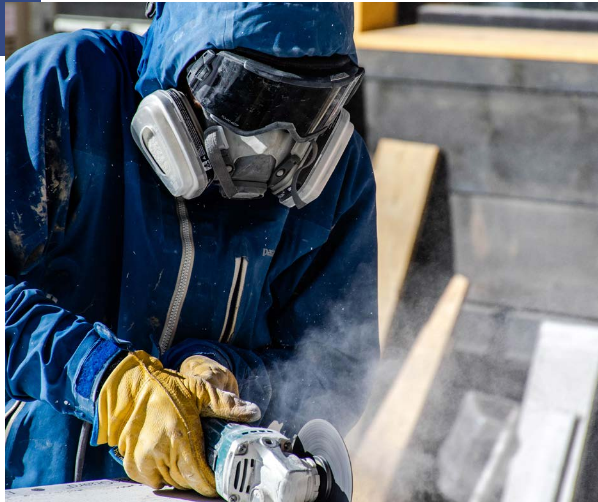
Our actual client Joe cutting cement board for the bathroom tiling.
